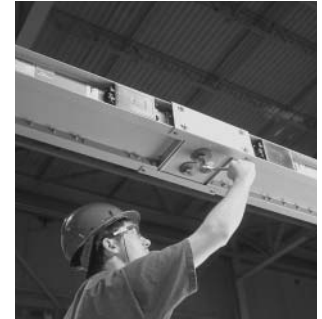
Typical Busway Installation (Torque Indicating Bolt)
